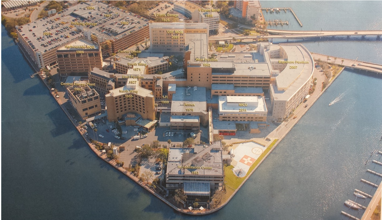
Figure 1. Tampa General Hospital Campus to be Served by Combined Heat & Power
